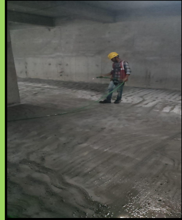
Curing for grade slab
