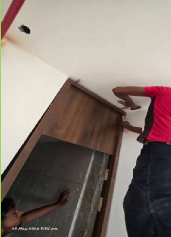
12th floor doors frame installation WIP
