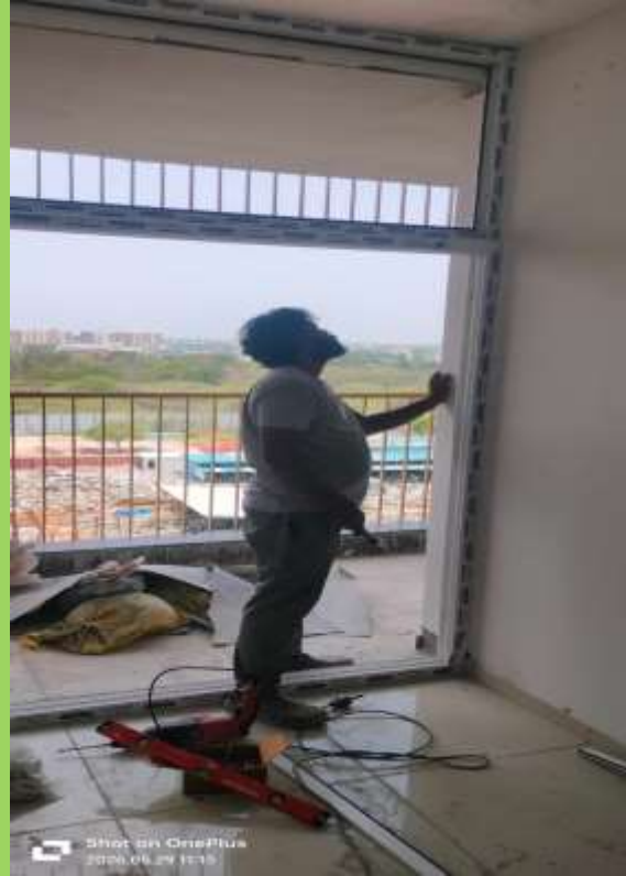
Flat - 830 UPVC windows & SLD fixing WIP
