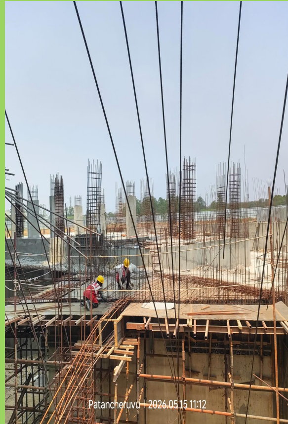
STP slab reinforcement WIP
