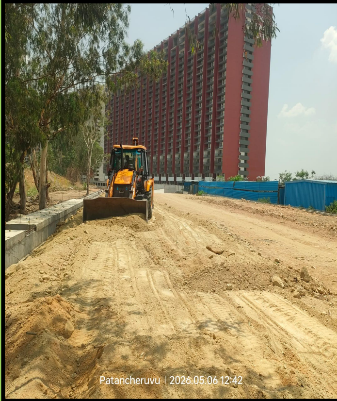
Soil Subgrade Soil preparation WIP
