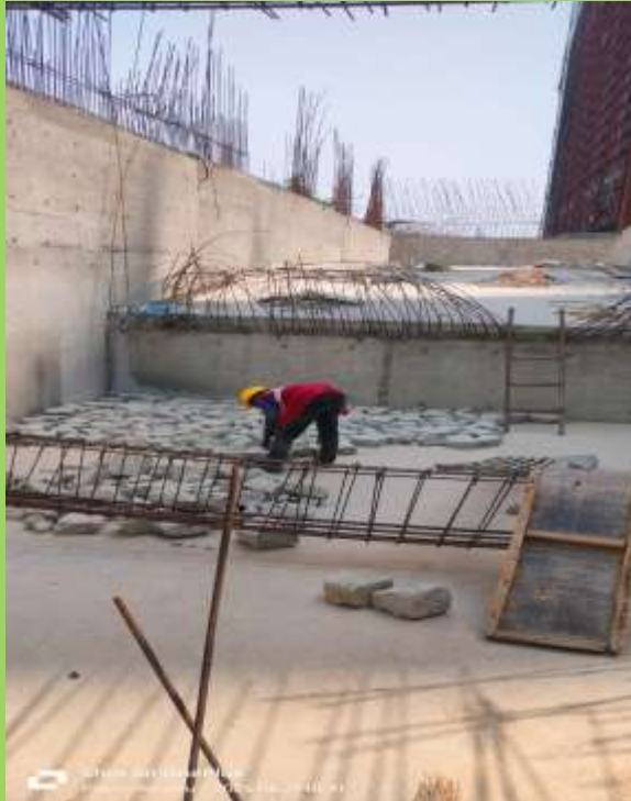
STP, Ramp area brick bat filling WIP
