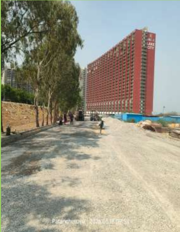
Main road GSB Dozing, levelling & compaction WIP
