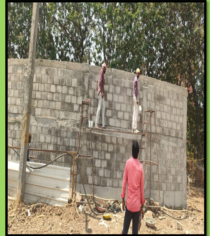
Curved wall fiber mesh fixing in wall joints.
