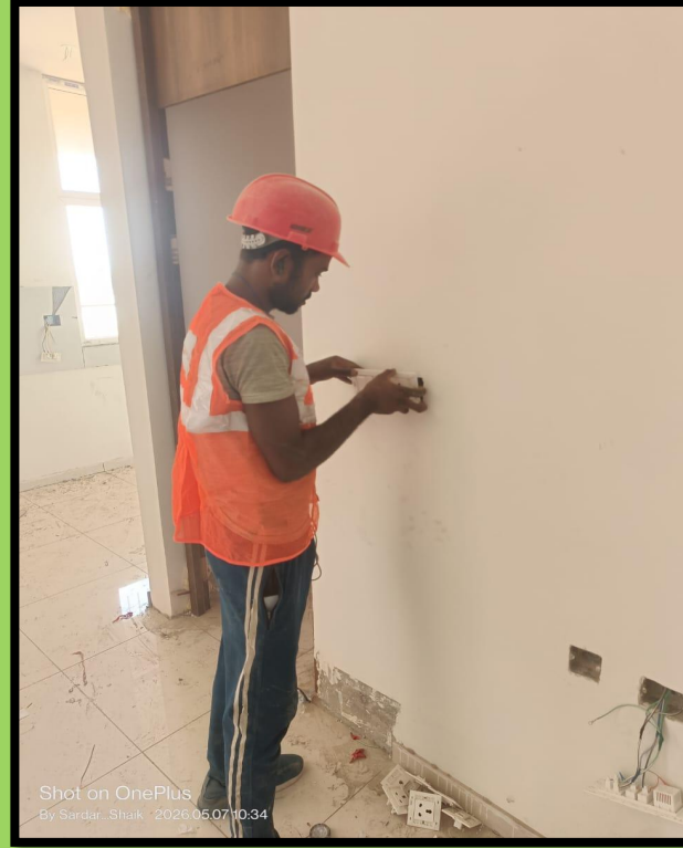
1305 & 1306 flats switchboard fixing WIP
