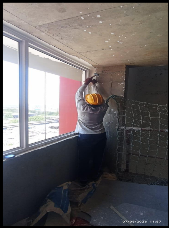
10th floor Lift lobby-01 Fixed windows installation WIP
