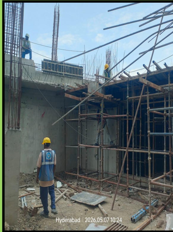
STP area shuttering WIP
