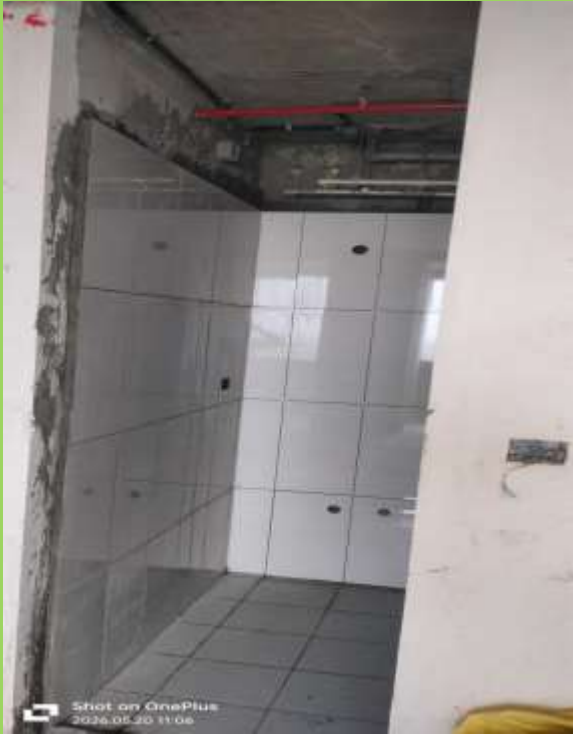
Flat -2119 toilet-02 wall dado and flooring work completed
