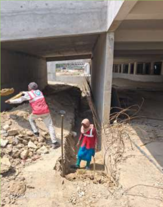
Earth ramp side drain excavation wip
