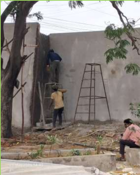
Curved wall back side plastering WIP
