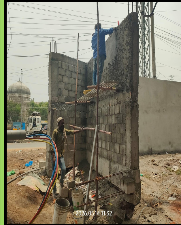
Curved wall plastering WIP
