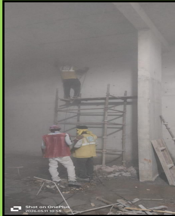
STP, Treated water tank walls buffing WIP
