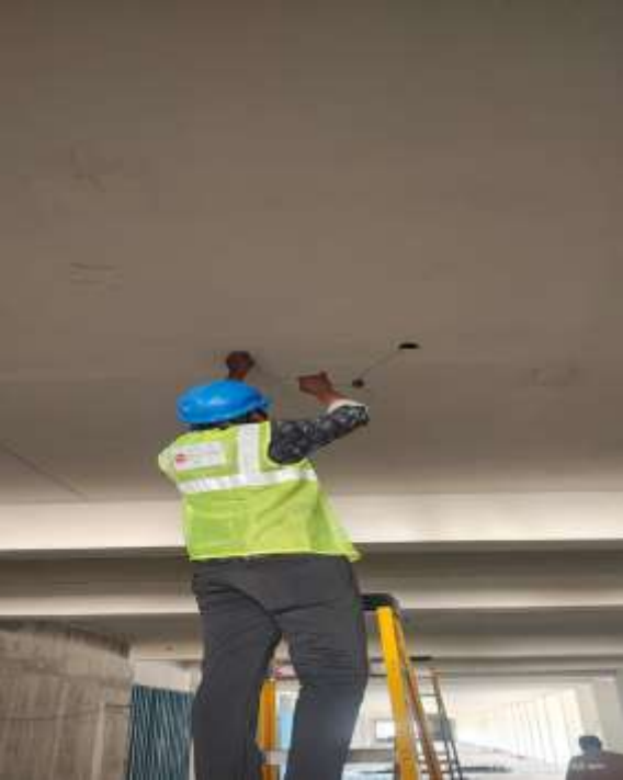
Basement -1 GI pulling WIP
