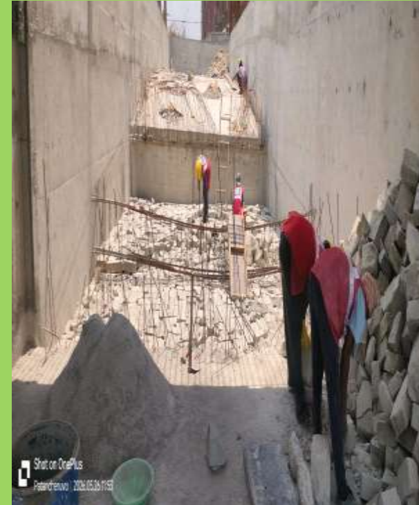
STP, Ramp area brickbat filling WIP
