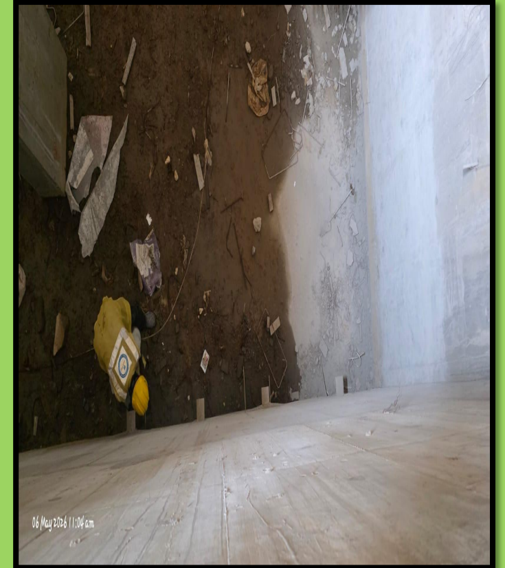
STP dead mortar chipping WIP
