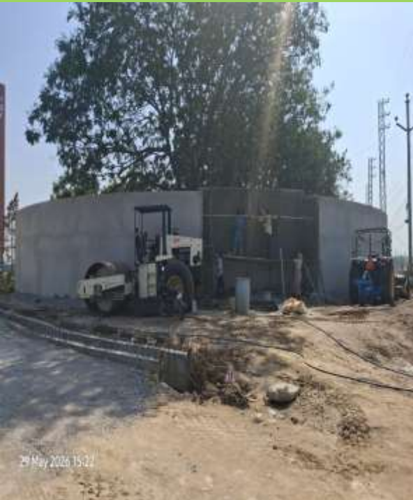
Curved wall front side plastering WIP
