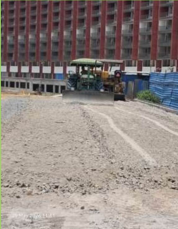
Entrance road WMM leveling WIP
