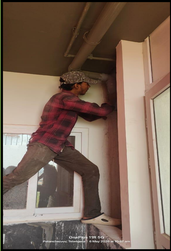
14th floor 6th flat kitchen shaft PVC piping WIP
