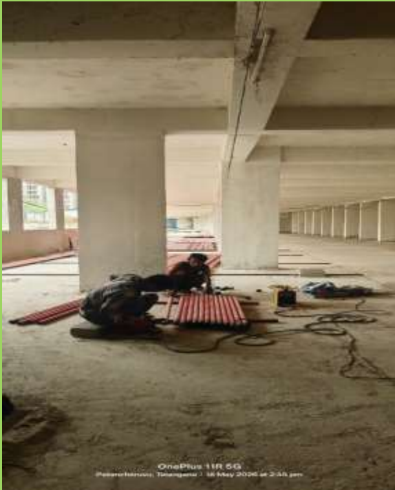
Basement - 1 fire fighting fabrication WIP
