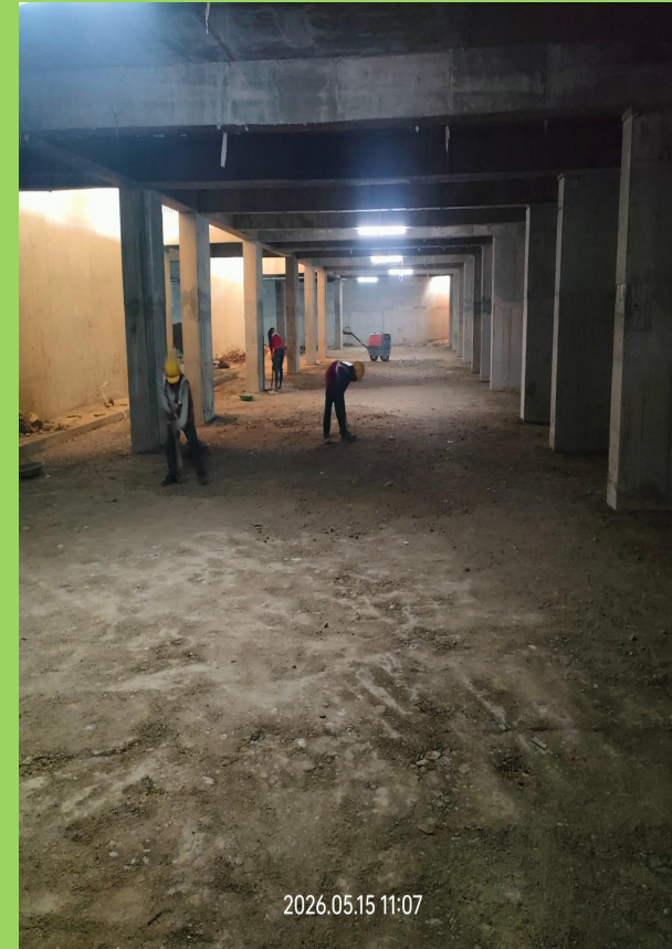
B-2 north side grade slab area soil dressing WIP
