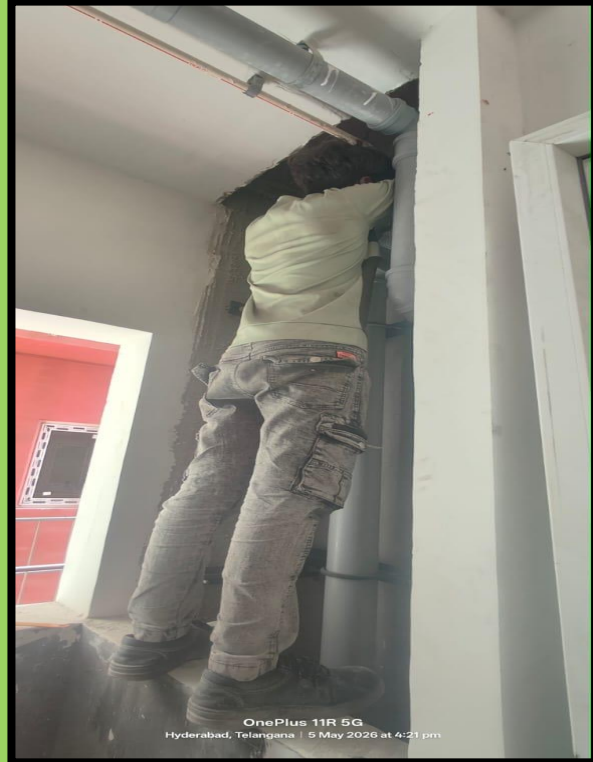
11th floor 23rd flat PVC piping WIP
