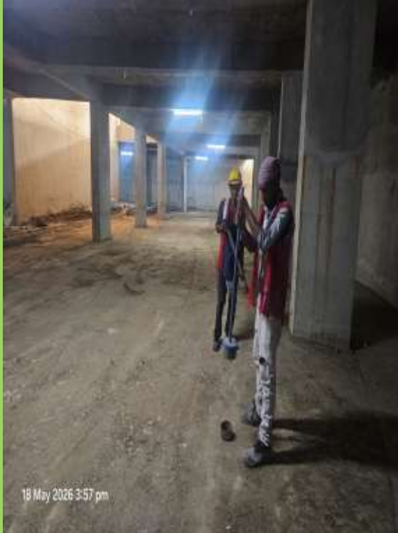
Tower-A B-2 Grade slab FDD test done for further works
