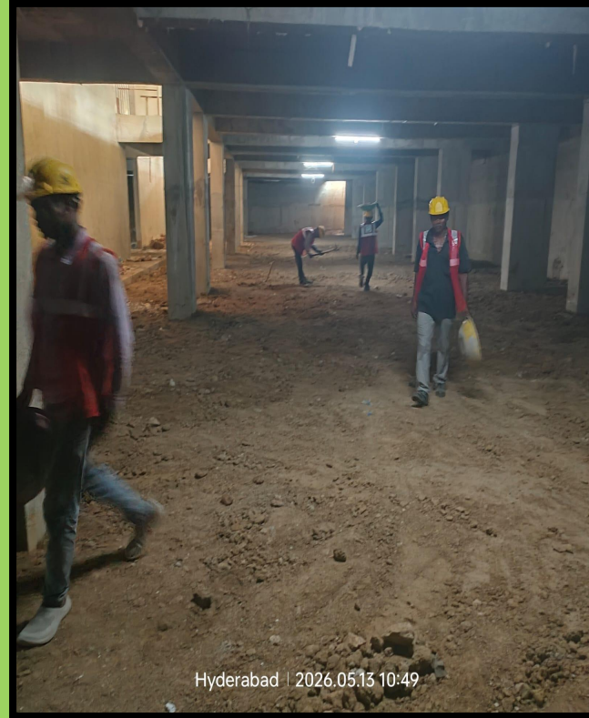
Tower-A B-2 north side grade slab area soil dressing WIP
