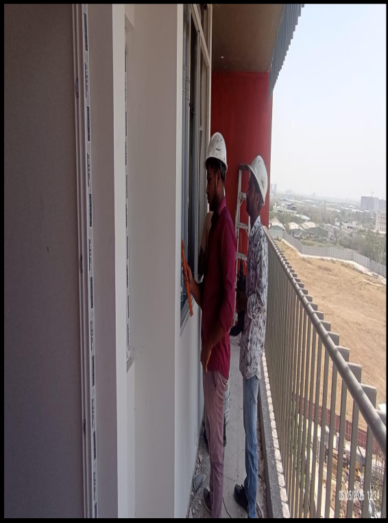
9th floor UPVC windows installation WIP
