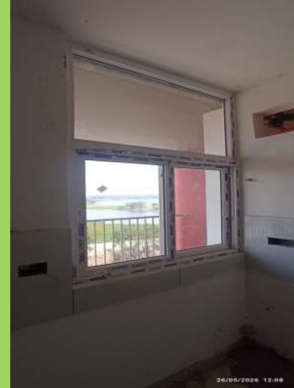
8 th Floor 1 to 5 flat Windows installation completed
