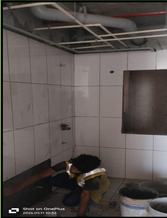
Flat 2120 wall dado and flooring WIP
