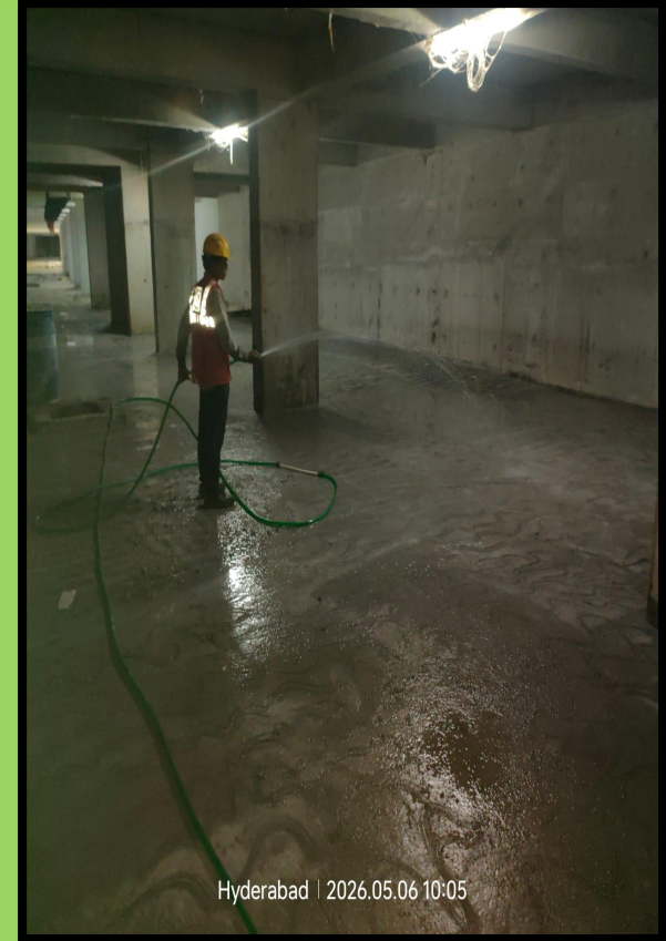
Curing for B-2 grade slab
