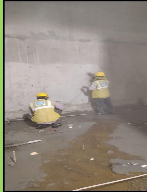
STP, Treated water tank walls buffing WIP
