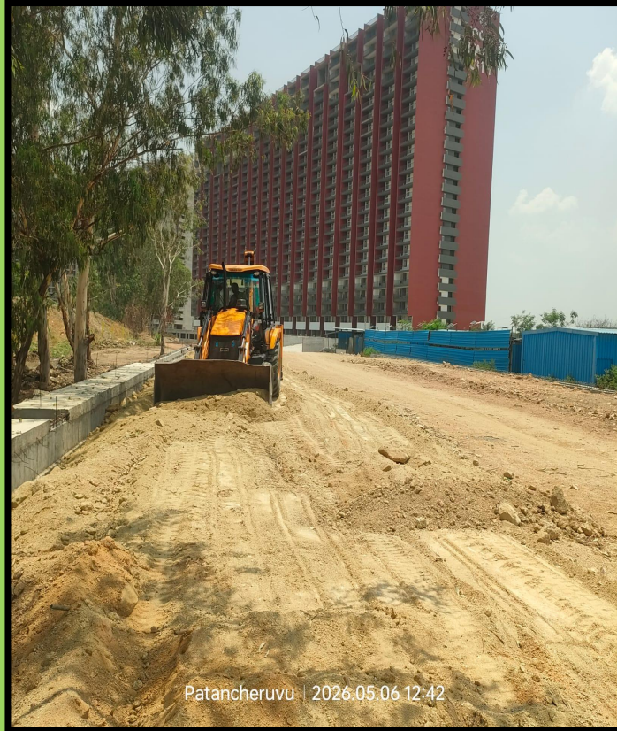
Soil Subgrade Soil preparation WIP
