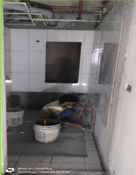
Flat - 2128 toilet-01 & 02 tile wall dado and flooring WIP
