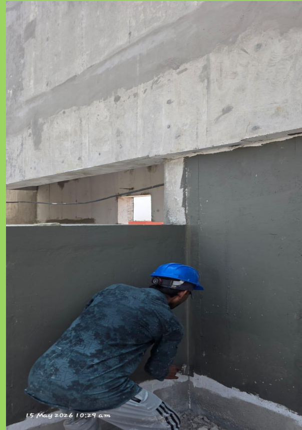
Terrace flat- 18 to 25 1st coat paint WIP
