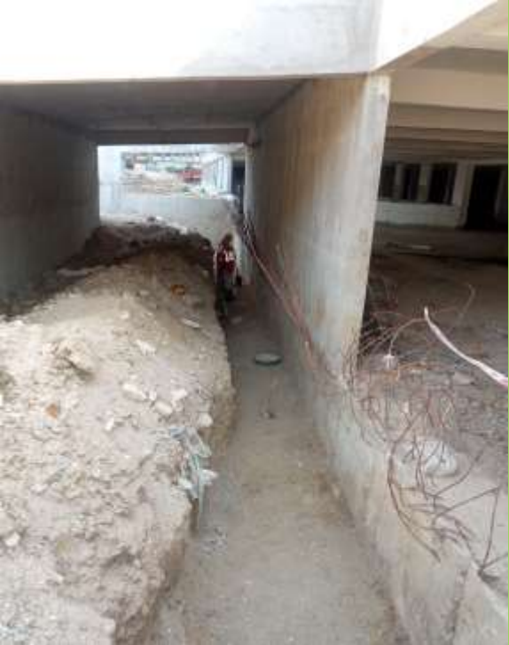
Entrance ramp drain excavation WIP
