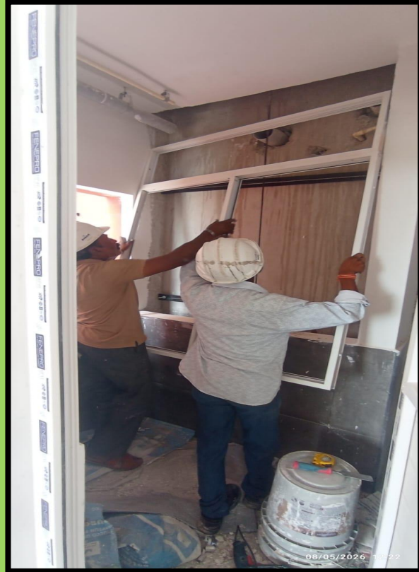
9th floor shaft doors frames installation WIP
