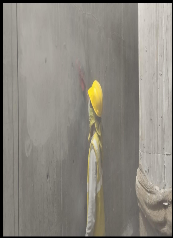
STP pump room buffing WIP
