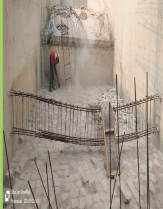
STP, Ramp area brickbat filling WIP
