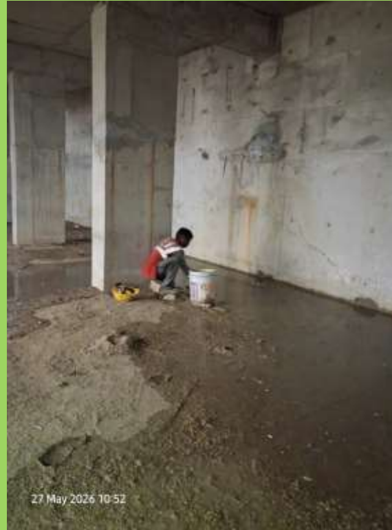
T-A grade slab cleaning WIP
