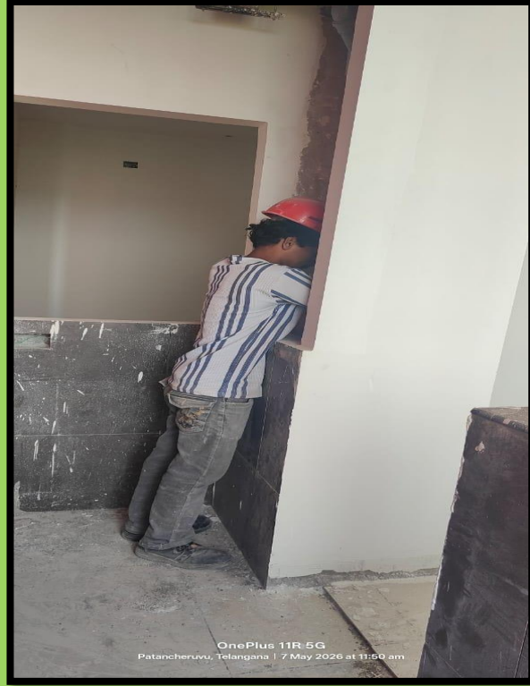
19th floor 5th flat PVC piping WIP
