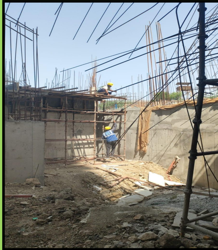
Stp area slab shuttering WIP
