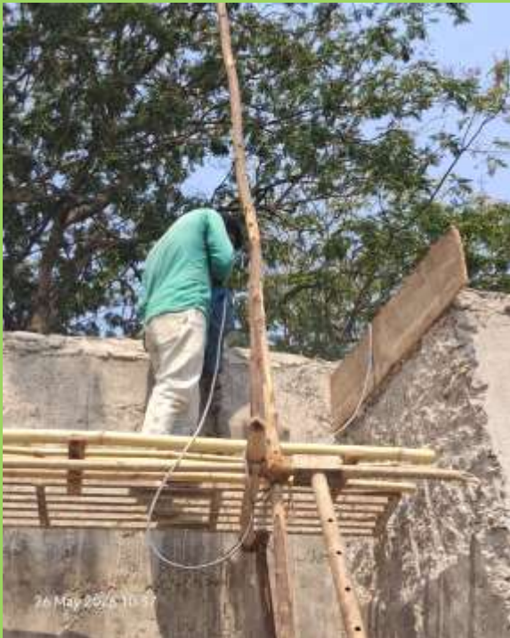
Curved wall front side chipping WIP
