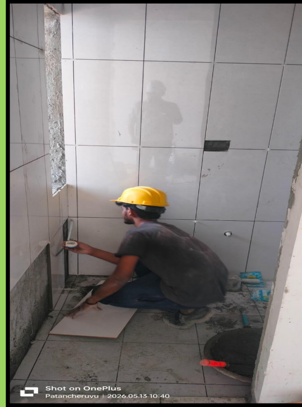
21st floor flat 23 , tile wall dado and flooring WIP
