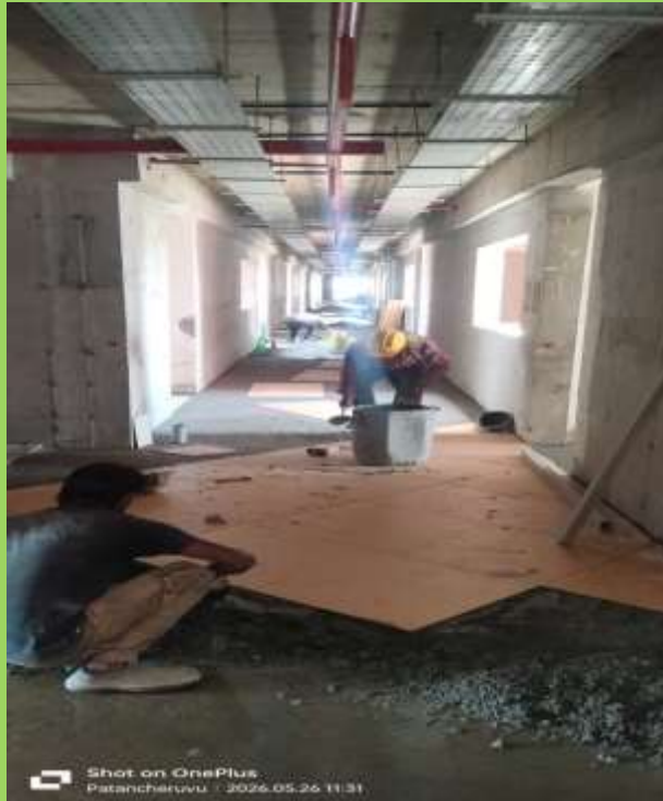
20th floor, corridor tile flooring WIP
