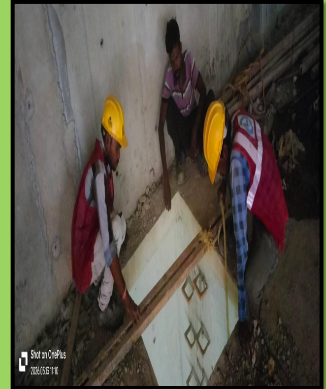
STP, Treated water debris removal and material shifting WIP
