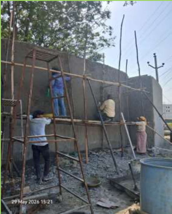
Curved wall front side plastering WIP
