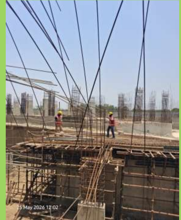
Stp side shuttering WIP
