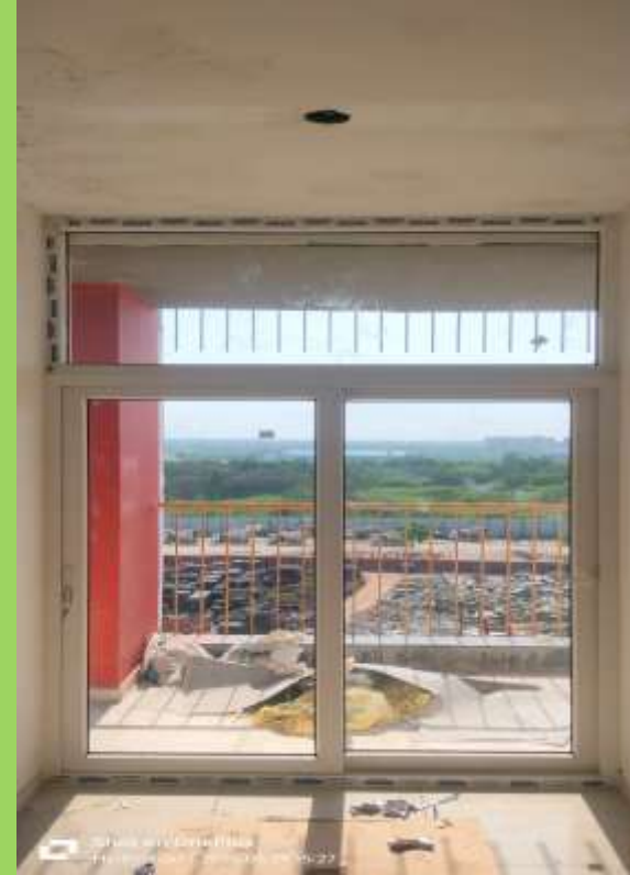
Flat - 830 Fixing of windows completed
