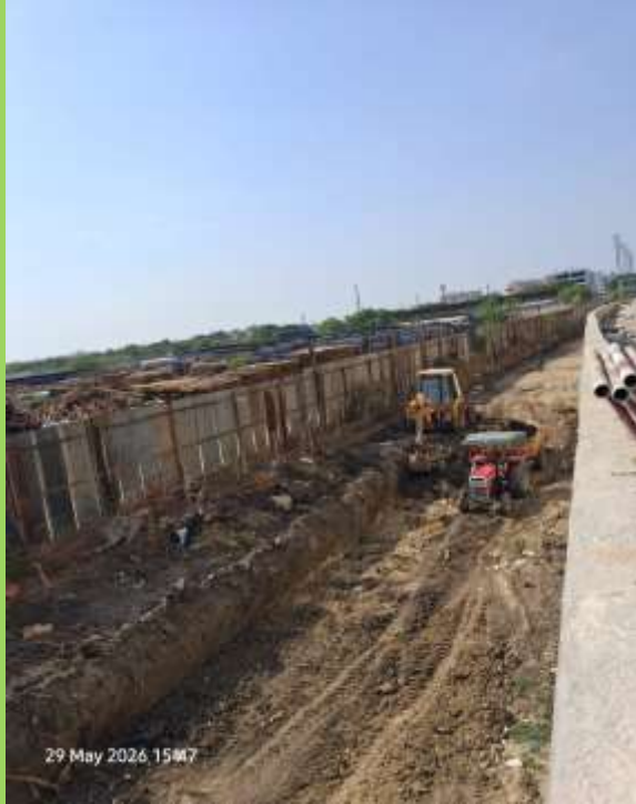
Transformer yard excavation work completed
