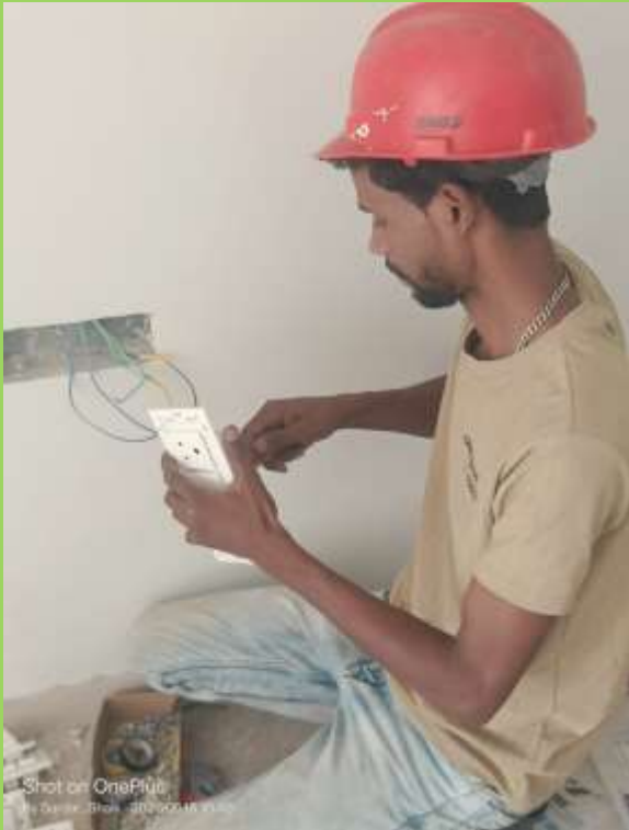
Flat-1311,1314 & 1315 Flats switchboard fixing WIP
