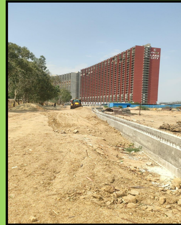
Storm water drains area back filling & levelling
