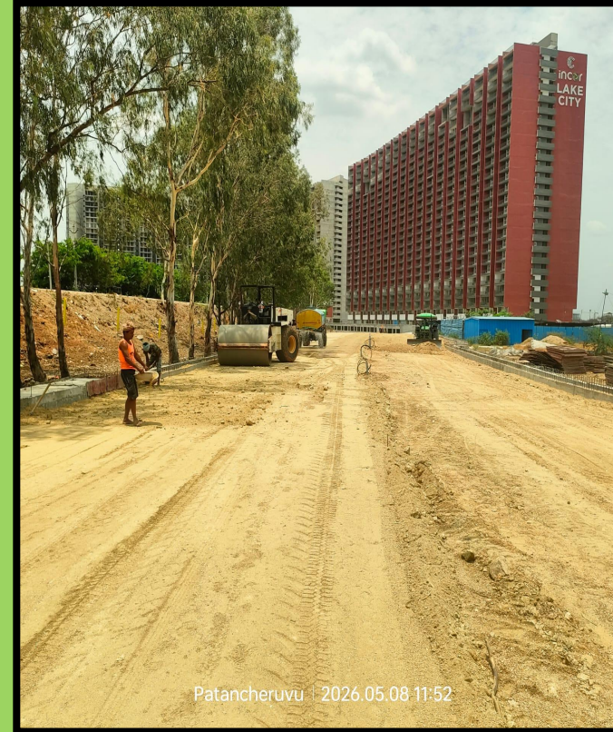
Water sprinkling for soil compaction WIP.
