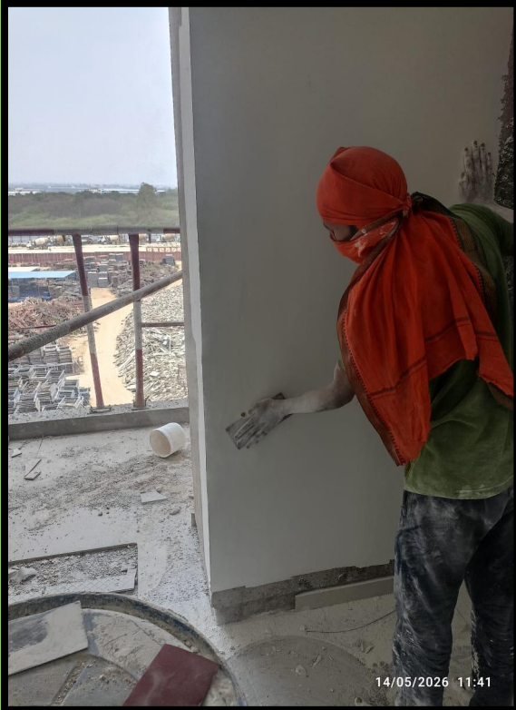
5th floor Flat-29 Sanding WIP
