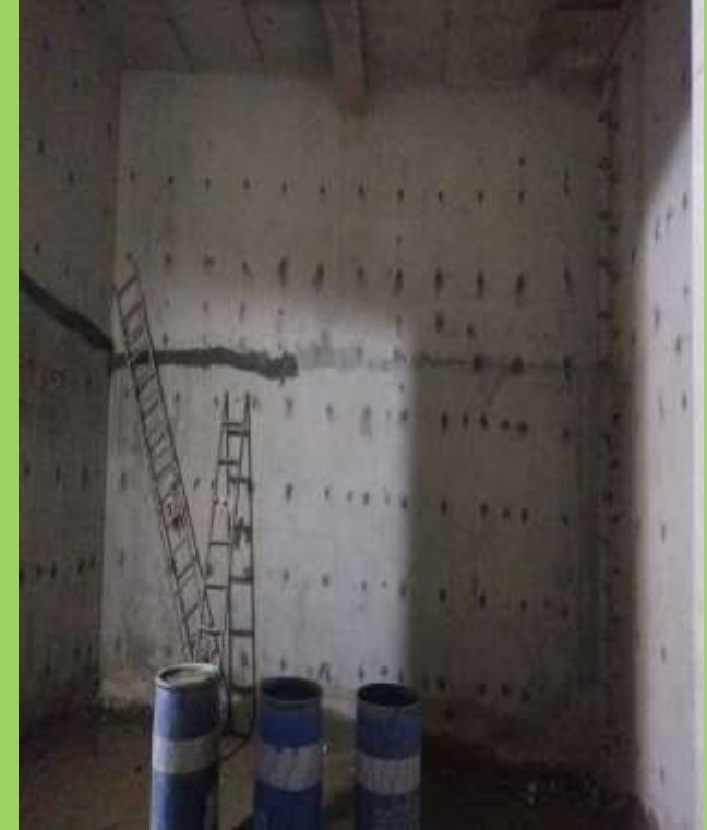
STP, Ultrafiltration tank debris removal and cleaning work completed
