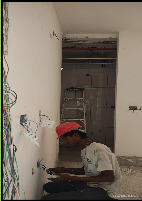
1307,06 switch board fixing and wiring WIP
