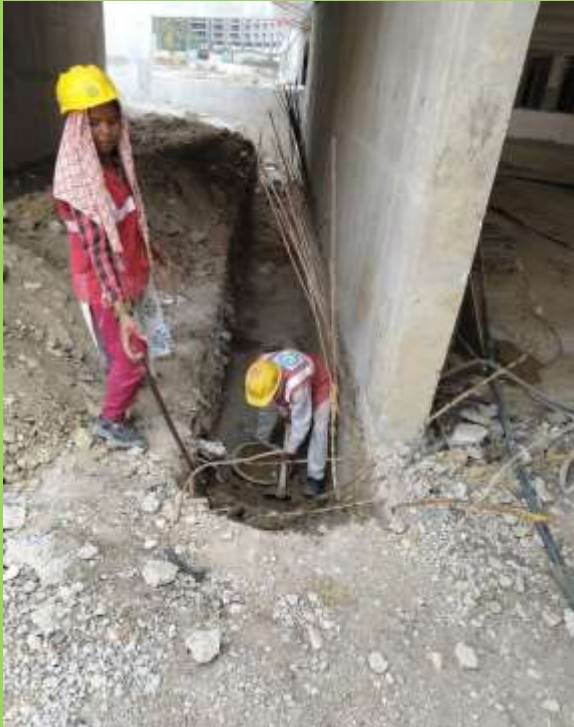
Earthen ramp area drain excavation work
