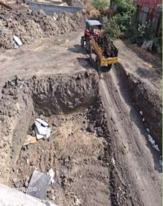
Transformer yard excavation work completed
