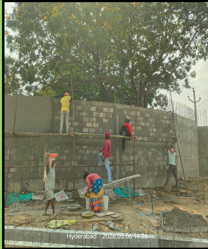
Curved wall plastering WIP
