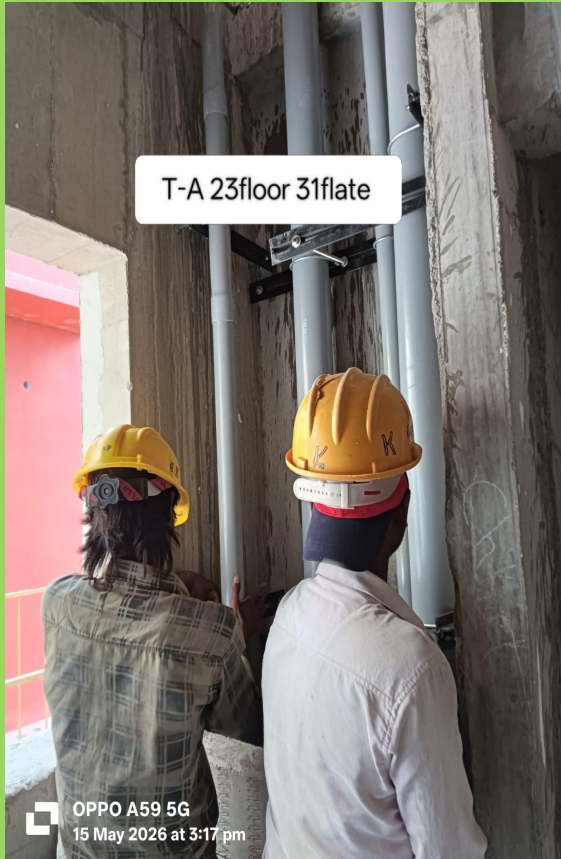
PVC & UPVC piping WIP
