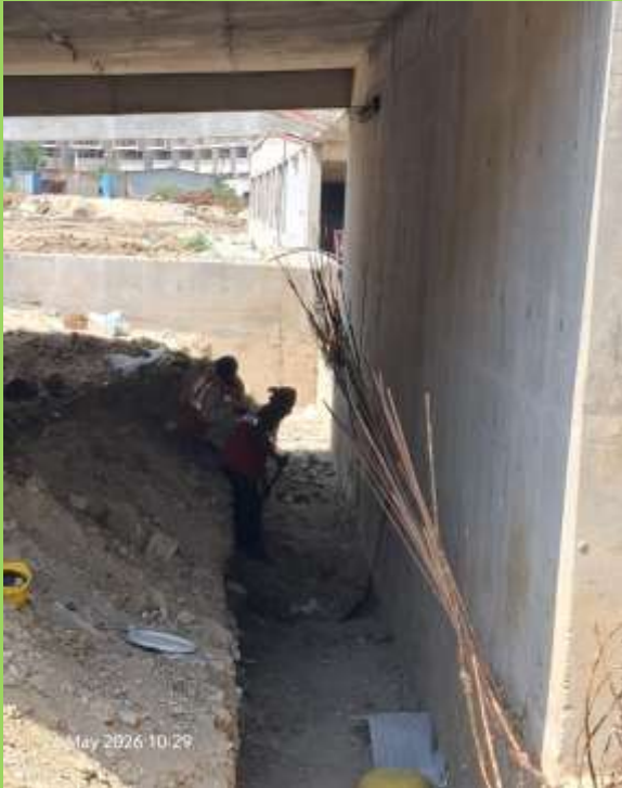
Earthen ramp drain excavation WIP
