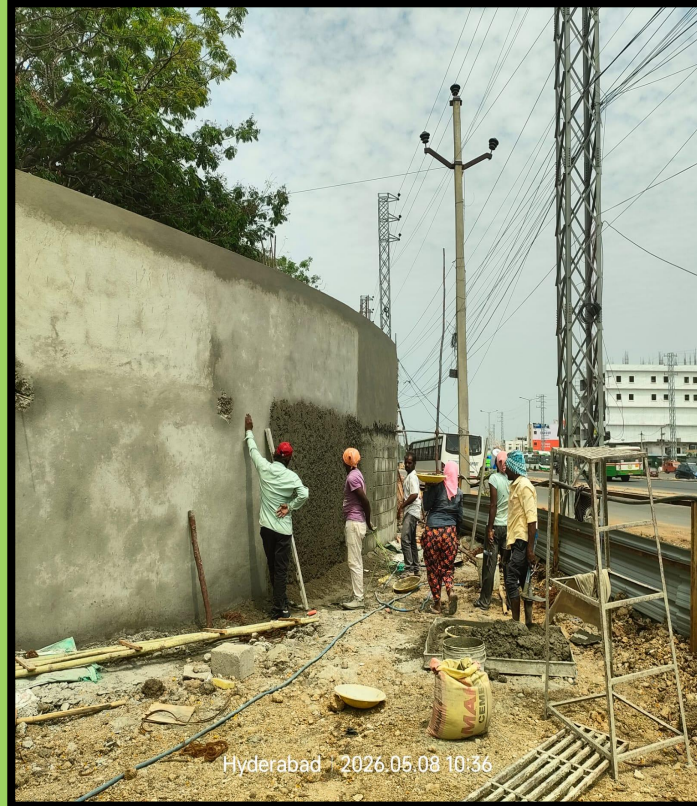
Curved wall plastering WIP
