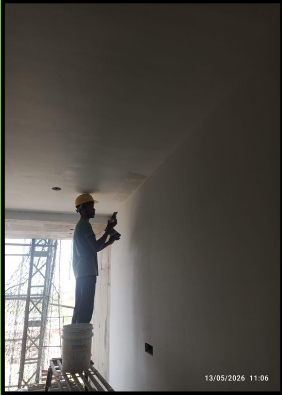
Flat-529 2nd coat Fine putty WIP
