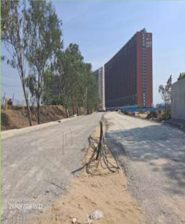
Entrance road WMM leveling WIP
