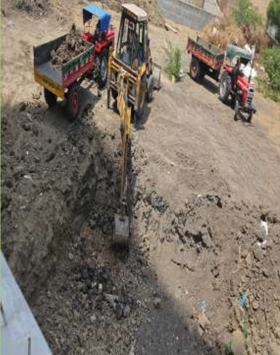
Transformer yard excavation WIP
