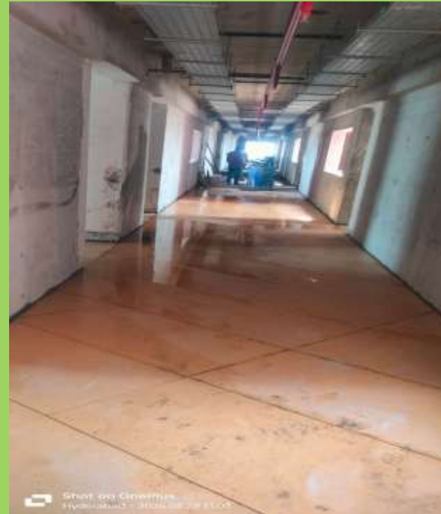
20th floor, corridor tile flooring WIP
