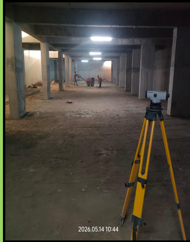
Tower-A B-2 north side grade slab area soil dressing compaction WIP
