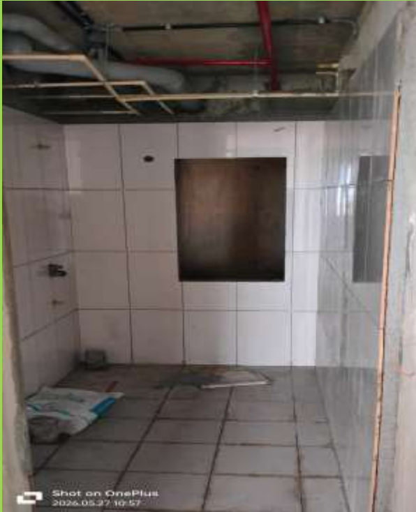
Flat - 2128 toilet-01 tile wall dado and flooring work completed
