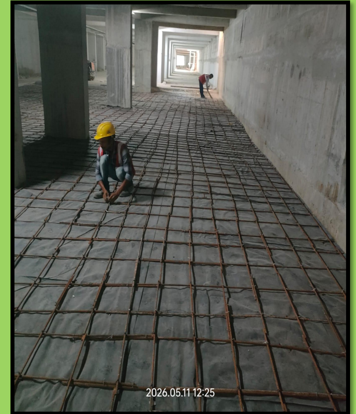
Tower-A B-2 west side grade slab casting WIP
