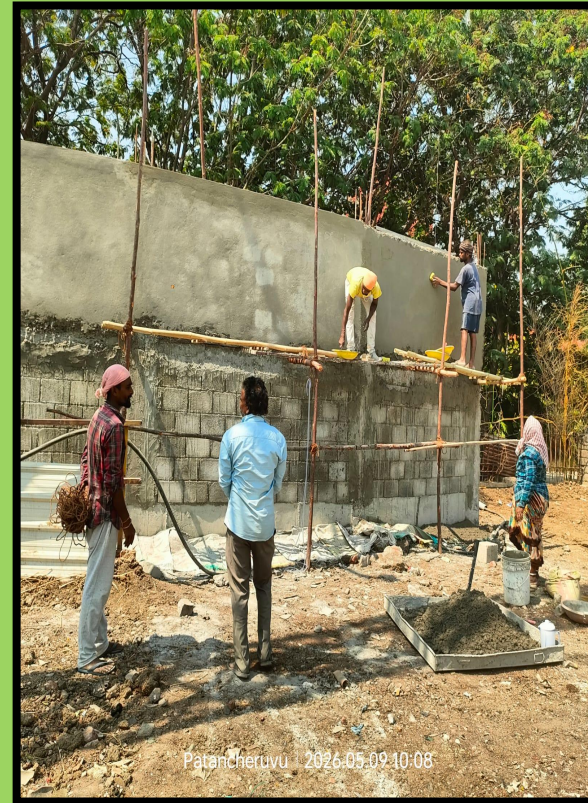
Curved wall plastering WIP
