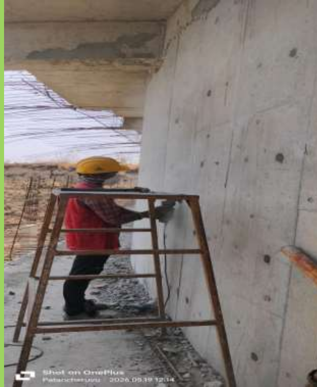
STP, outer face, south side walls buffing WIP
