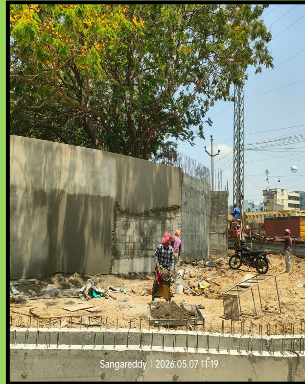
Curved wall plastering WIP
