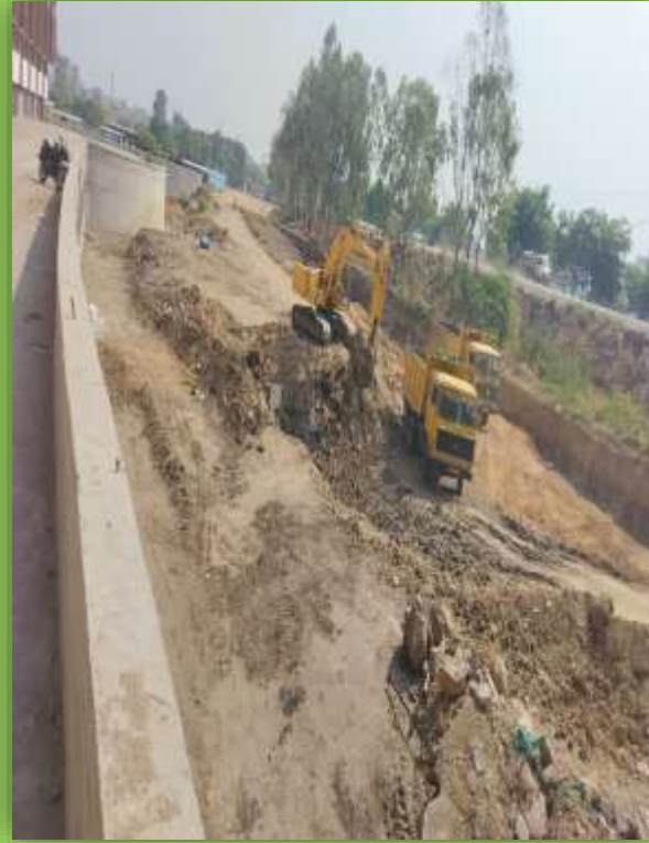
Existing road excavation work in progress at tower -A
