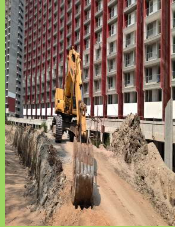
Excavation work at Tower A
