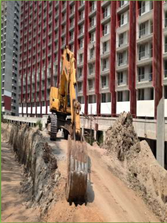
Excavation work at Tower A
