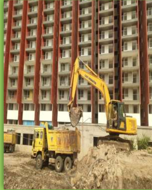
Excavation work at Tower A
